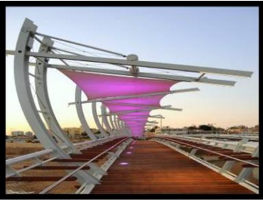
Pipes Bridge in Be'er Sheva
